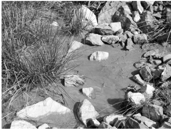
Red ooze from Lot 21 leaching into Shawnigan Creek
